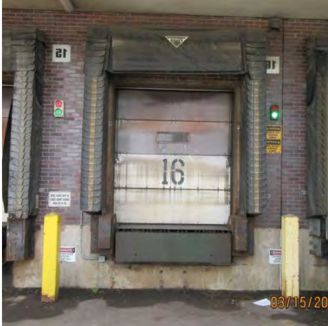
DOOR 16 Remove Existing Red/Green Light System
