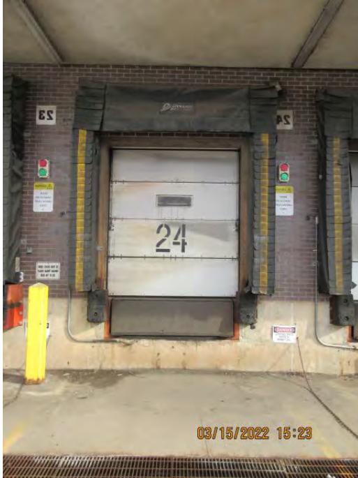
DOOR 24 Remove Existing Red/Green Light System
