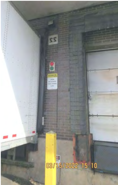
DOOR 22 Remove Existing Red/Green Light System
