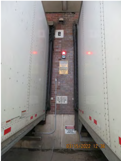
DOOR 9 Remove Existing Red/Green Light System
