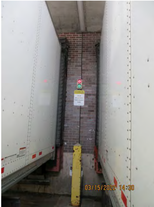
DOOR 19 Remove Existing Red/Green Light System
