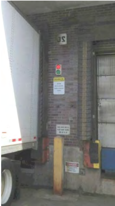
DOOR 20 Remove Existing Red/Green Light System
