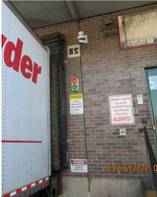
DOOR 28 Remove Existing Red/Green Light System
