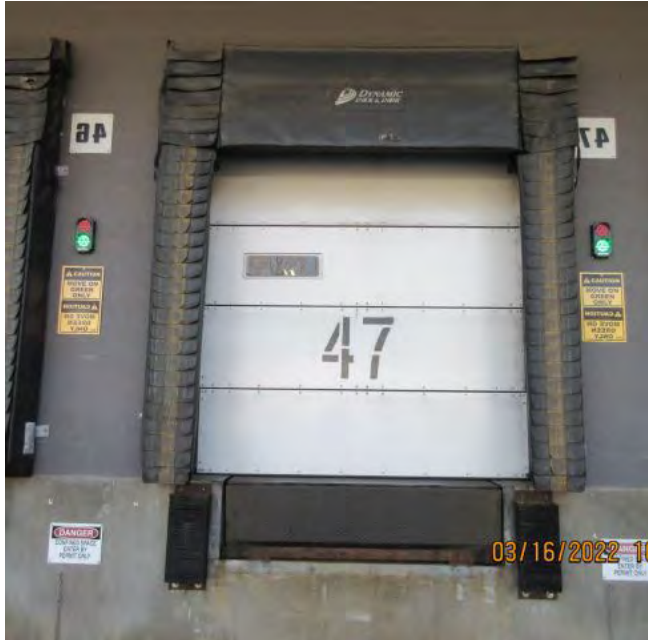
DOOR 47 Remove Existing Red/Green Light System
