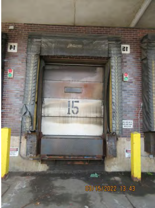
DOOR 15 Remove Existing Red/Green Light System
