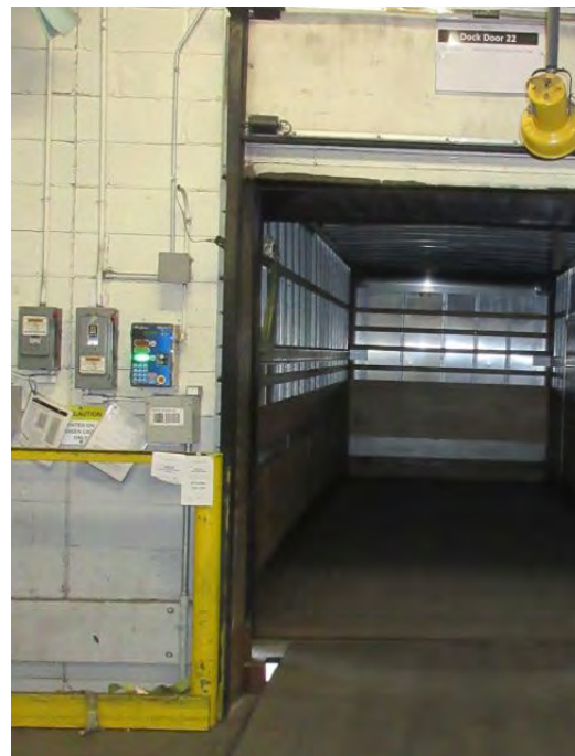
Existing Red/Green Light Controls, Left side of DOOR 22
