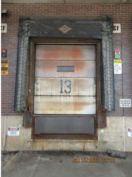
DOOR 13 Remove Existing Red/Green Light System
