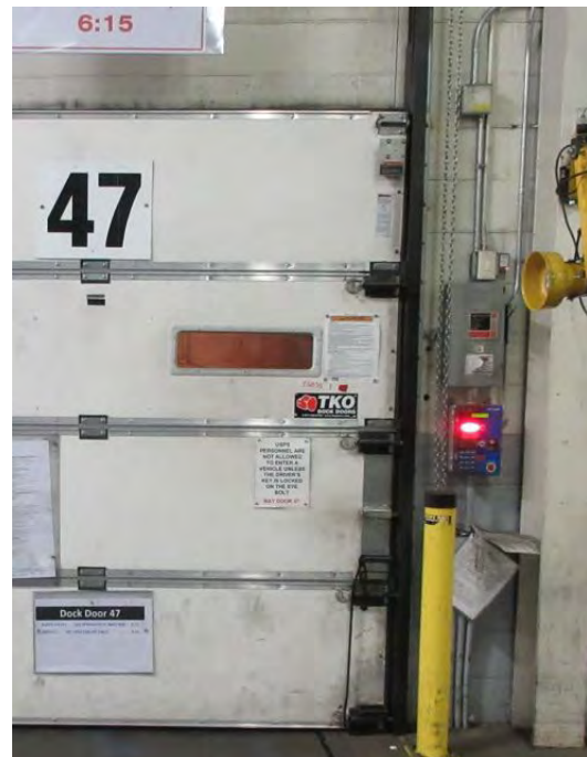
Existing Red/Green Light Controls, Right side of DOOR 47
