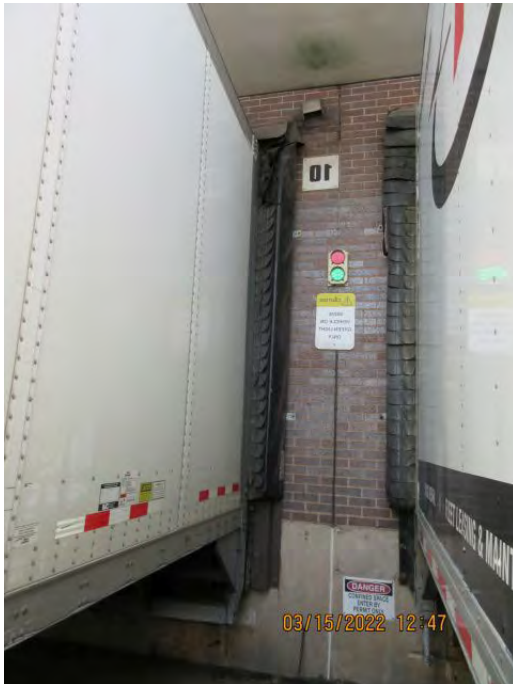
DOOR 10 Remove Existing Red/Green Light System
