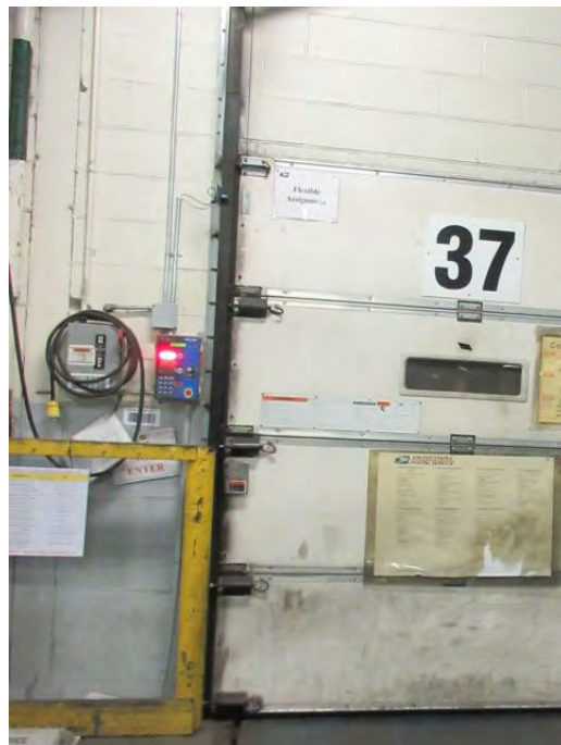
Existing Red/Green Light Controls, Left side of DOOR 37
