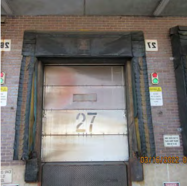
DOOR 27 Remove Existing Red/Green Light System
