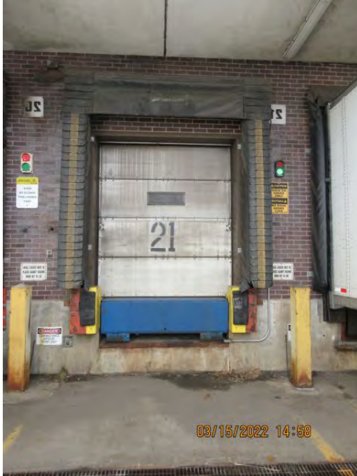
DOOR 20 Remove Existing Red/Green Light System
