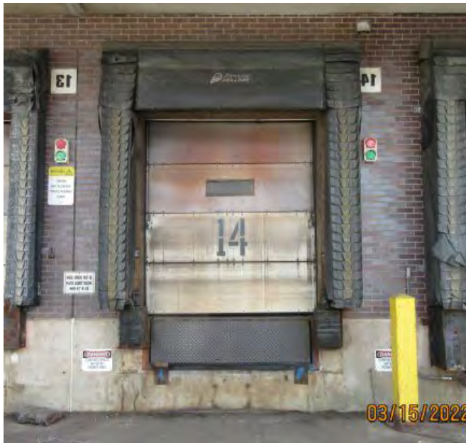
DOOR 14 Remove Existing Red/Green Light System
