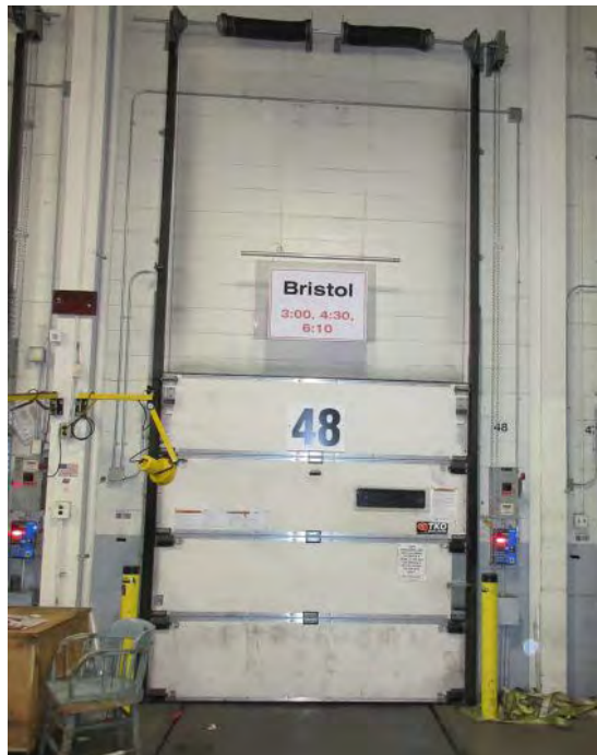
DOOR 48 Remove Existing Red/Green Light System
