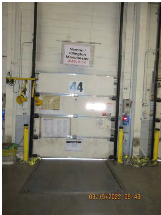
DOOR 44 Remove Existing Red/Green Light System
