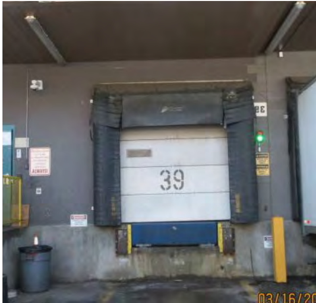
DOOR 39 Remove Existing Red/Green Light System
