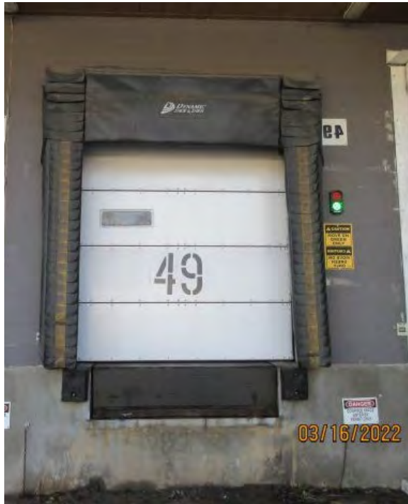
DOOR 49 Remove Existing Red/Green Light System
