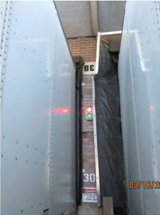
DOOR 30 Remove Existing Red/Green Light System
