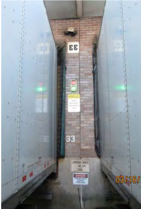
DOOR 33 Remove Existing Red/Green Light System
