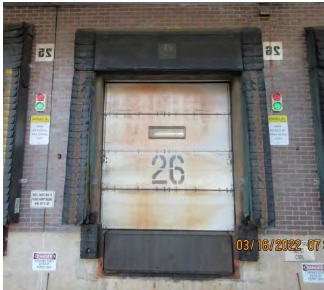
DOOR 26 Remove Existing Red/Green Light System
