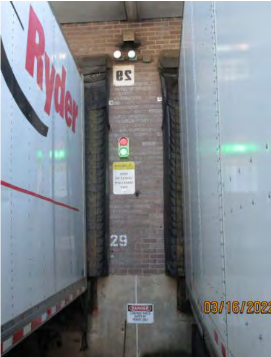
DOOR 29 Remove Existing Red/Green Light System
