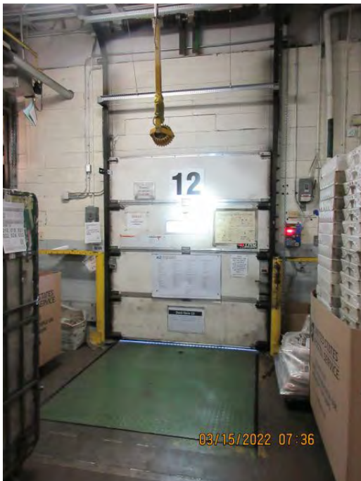
DOOR 12 Remove Existing Red/Green Light System
