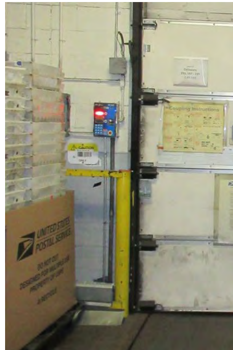
Existing Red/Green Light Controls, Left side of DOOR 10
