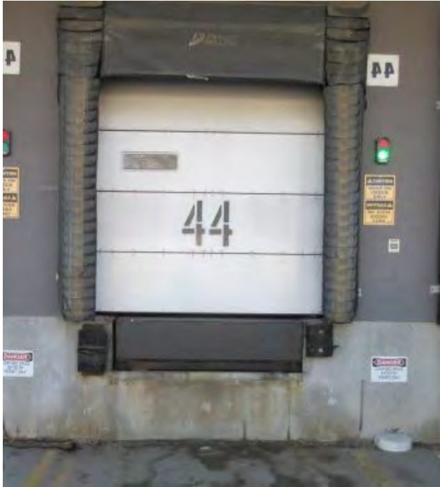
DOOR 44 Install Star 4 Truck Restraint
