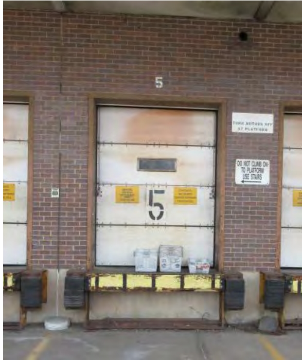
DOOR 5 Install Kelley Dock Communication System
