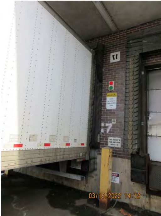
DOOR 17 Remove Existing Red/Green Light System
