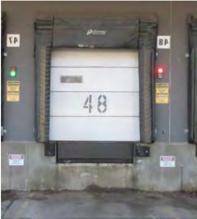
DOOR 48 Install Star 4 Truck Restraint
