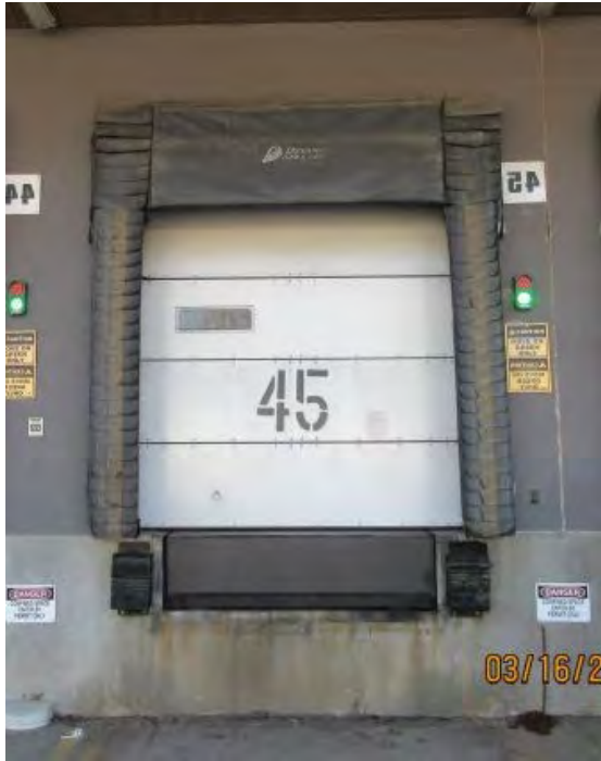
DOOR 45 Install Star 4 Truck Restraint
