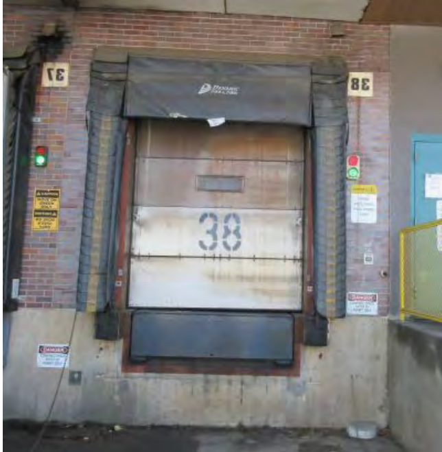
DOOR 38 Remove Existing Red/Green Light System
