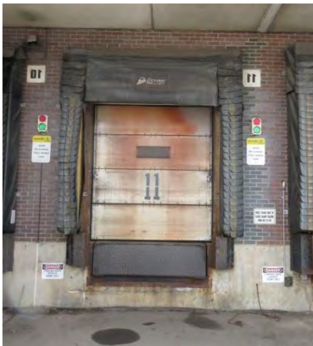
DOOR 11 Remove Existing Red/Green Light System
