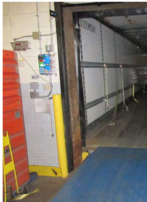
Existing Red/Green Light Controls, Left side of DOOR 9
