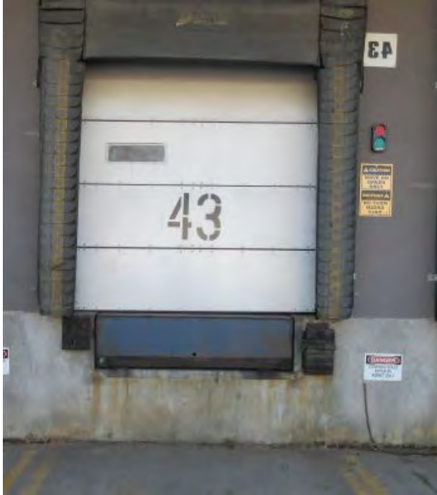
DOOR 43 Install Star 4 Truck Restraint
