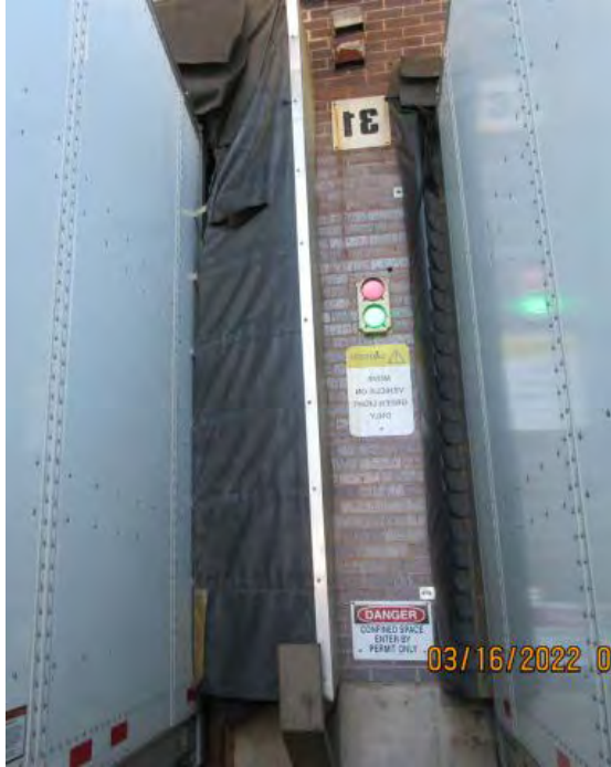
DOOR 31 Remove Existing Red/Green Light System
