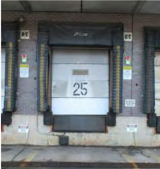
DOOR 25 Remove Existing Red/Green Light System
