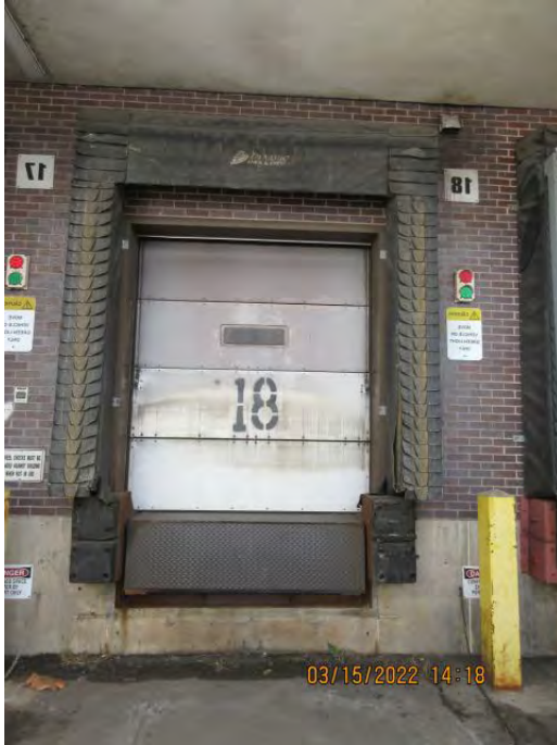
DOOR 18 Remove Existing Red/Green Light System
