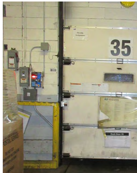
Existing Red/Green Light Controls, Left side of DOOR 35
