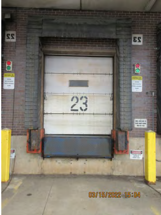
DOOR 23 Remove Existing Red/Green Light System
