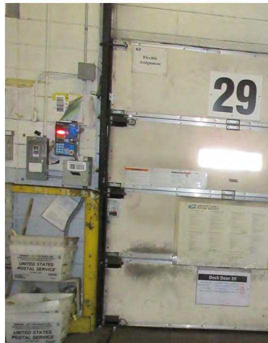
Existing Red/Green Light Controls, Left side of DOOR 29
