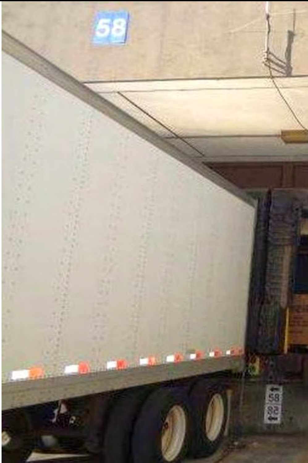
DOOR 58 Install Star 4 Truck Restraint W/ Cantilever Mounting Bracket along with Kelley Dock Control Box Mounted to Stanchion
