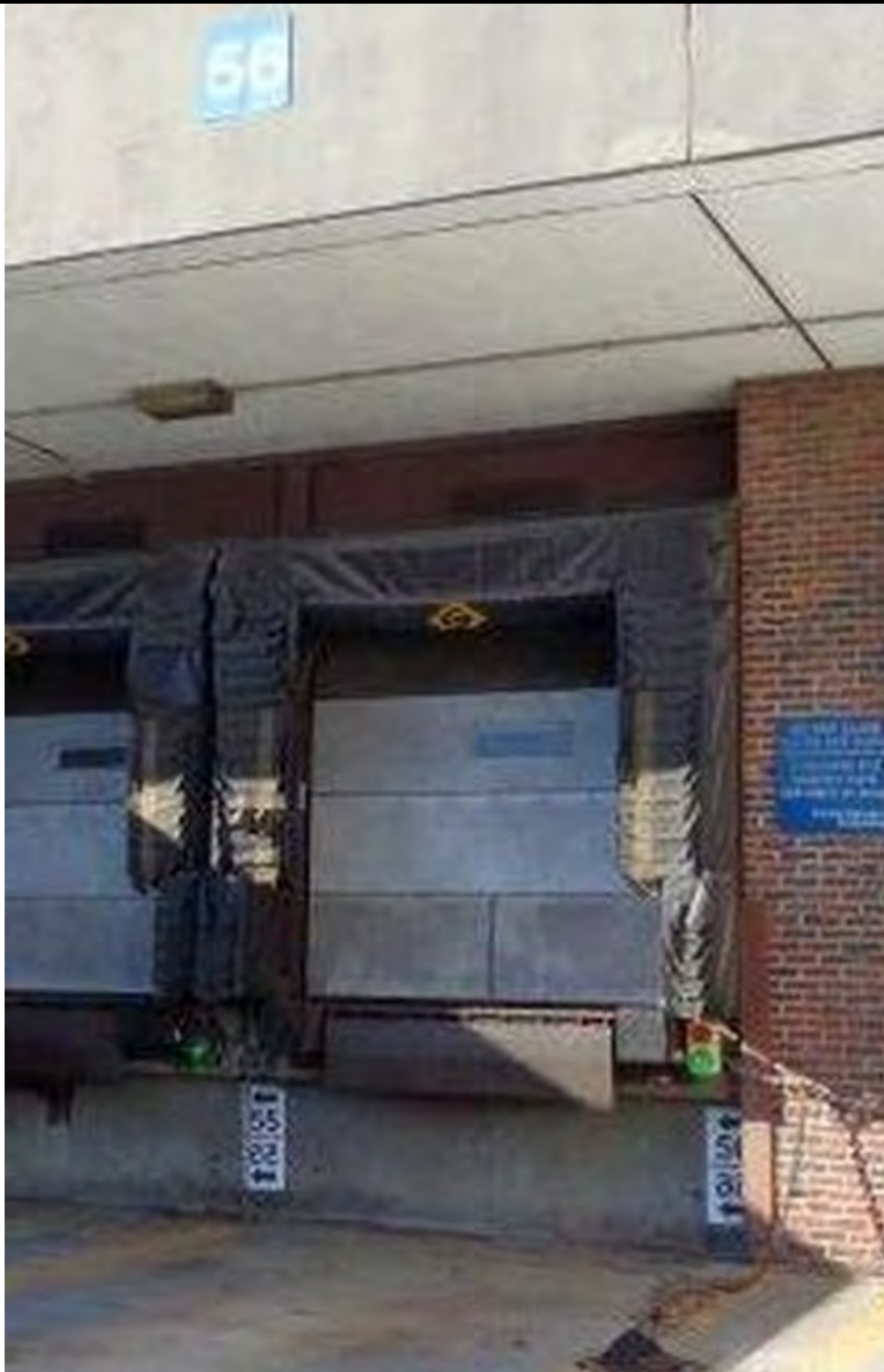
DOOR 56 Install Star 4 Truck Restraint W/ Cantilever Mounting Bracket along with Kelley Dock Control Box Mounted to Stanchion
