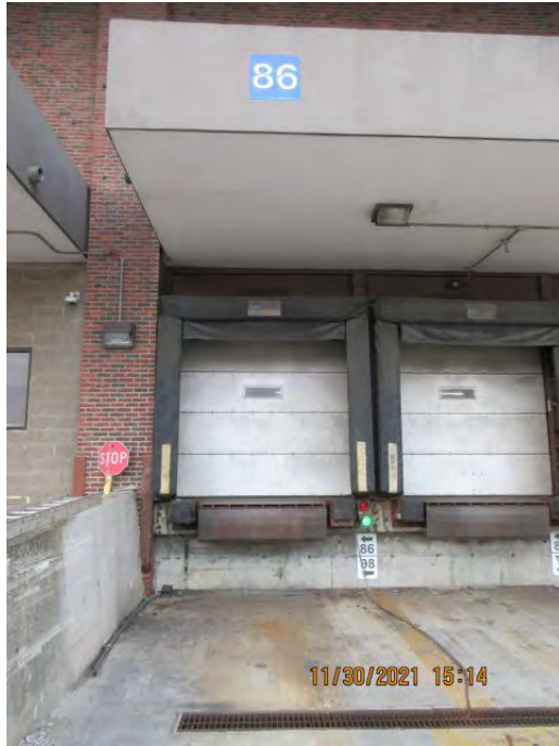
DOOR 86 Install Star 4 Truck Restraint W/ Cantilever Mounting Bracket
