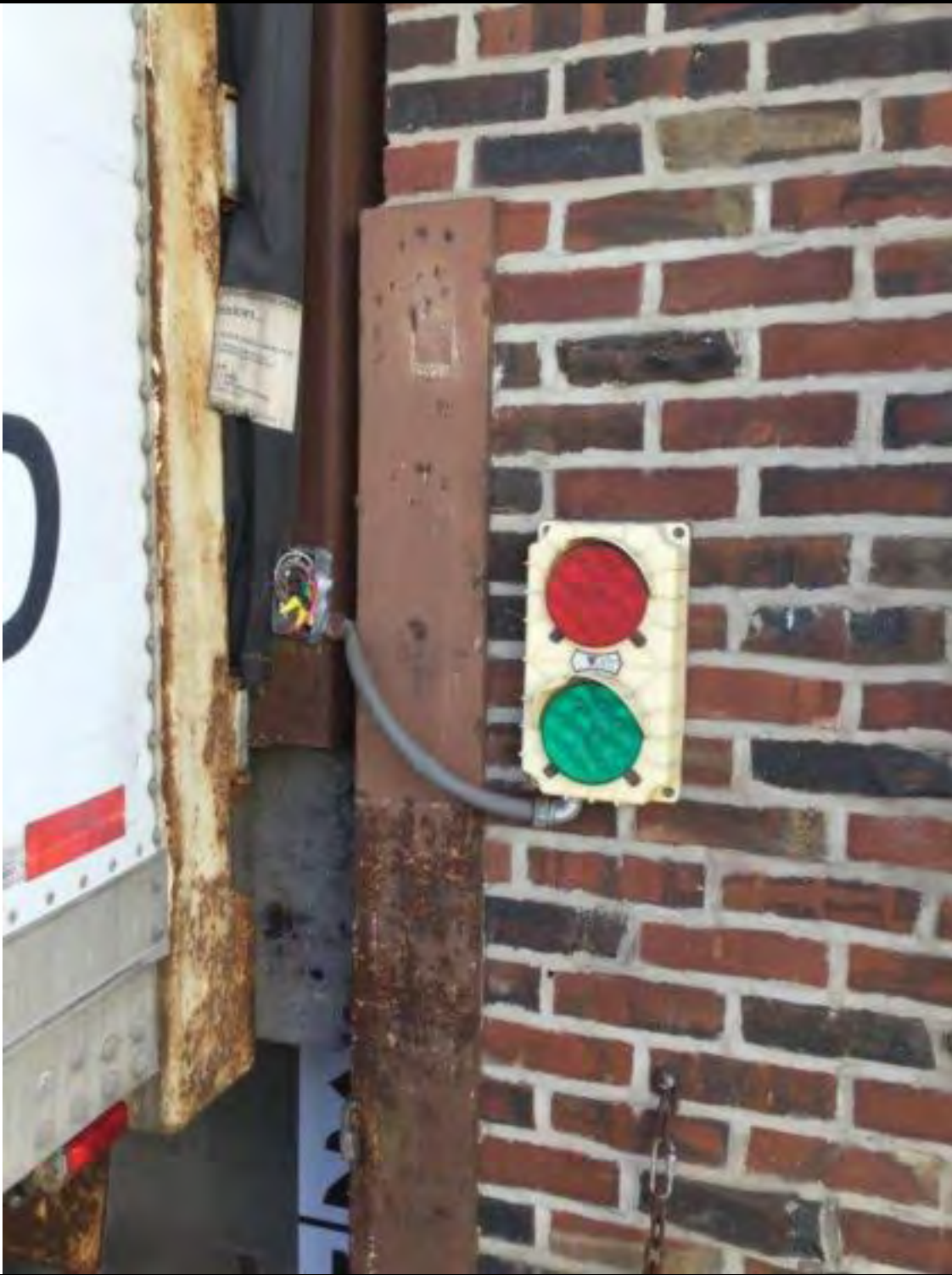
DOOR 24 Install Star 4 Truck Restraint W/ Cantilever Mounting Bracket
