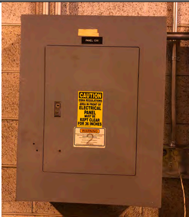
OLD DOORS 1-12 Panel C1X1 Add New 1 Pole 20A Circuit Breaker (1 for every 4 Doors)
