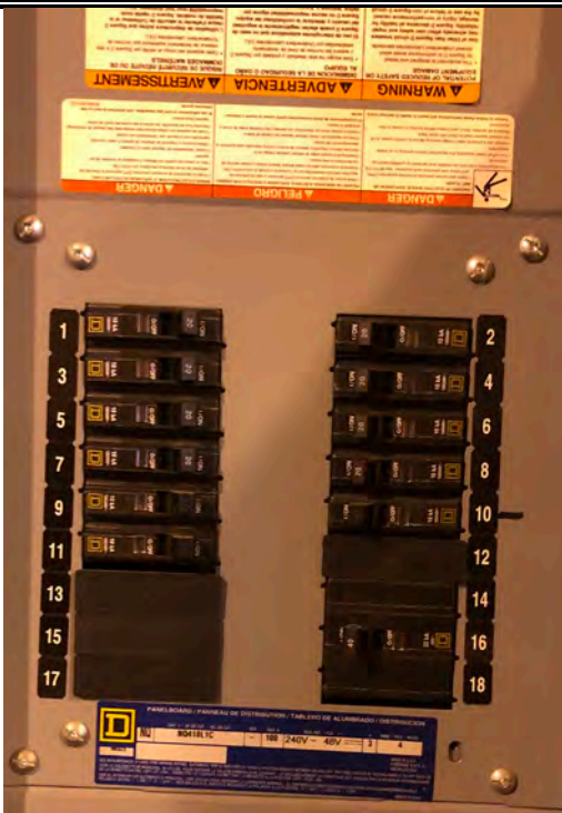
OLD DOORS 1-12 Panel C1X1 (connect no more than 4 TRS per circuit breaker)
