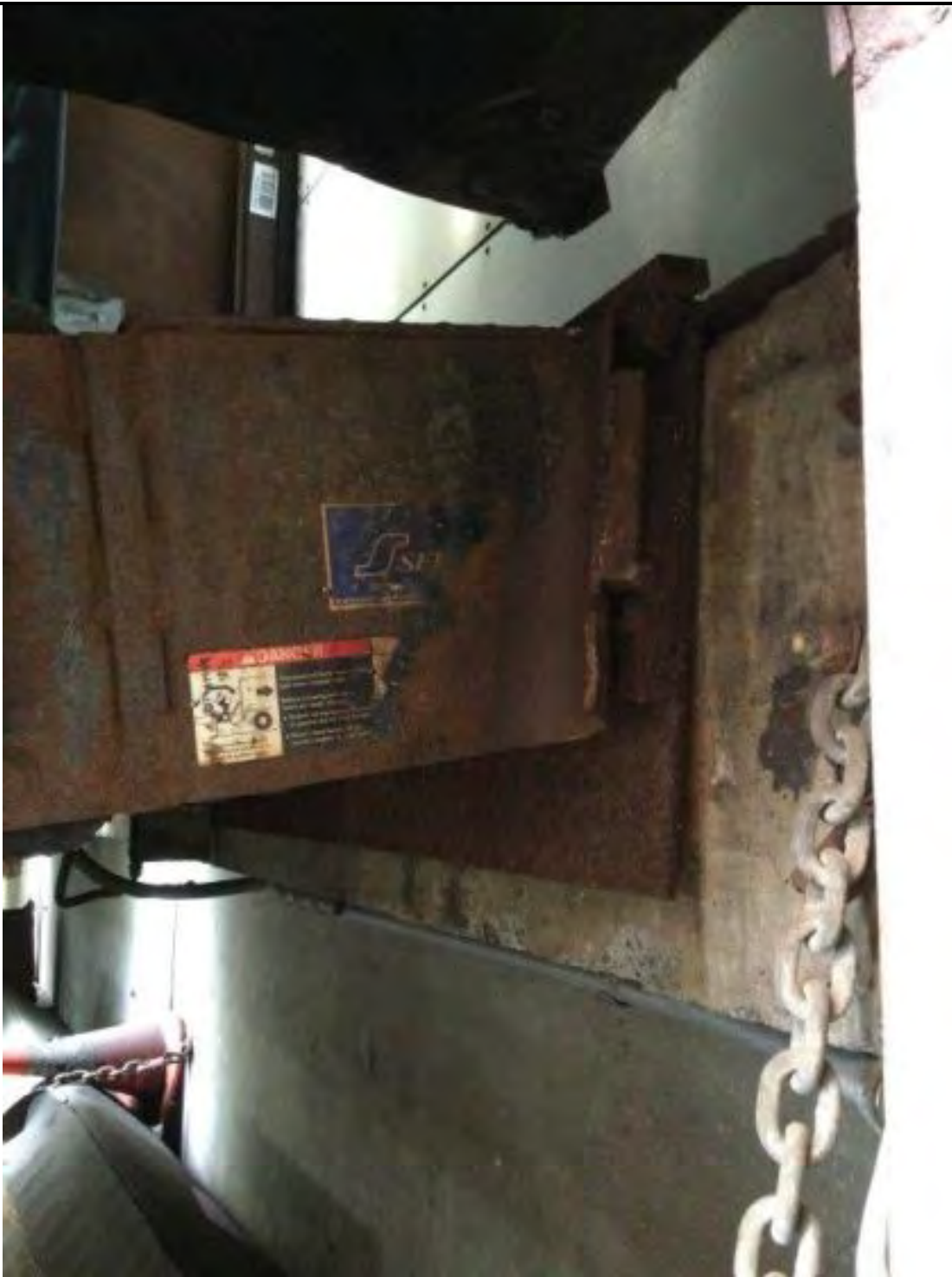
DOOR 45 Install Star 4 Truck Restraint W/ Cantilever Mounting Bracket, Provide and Replace Rubber Dock Bumper
