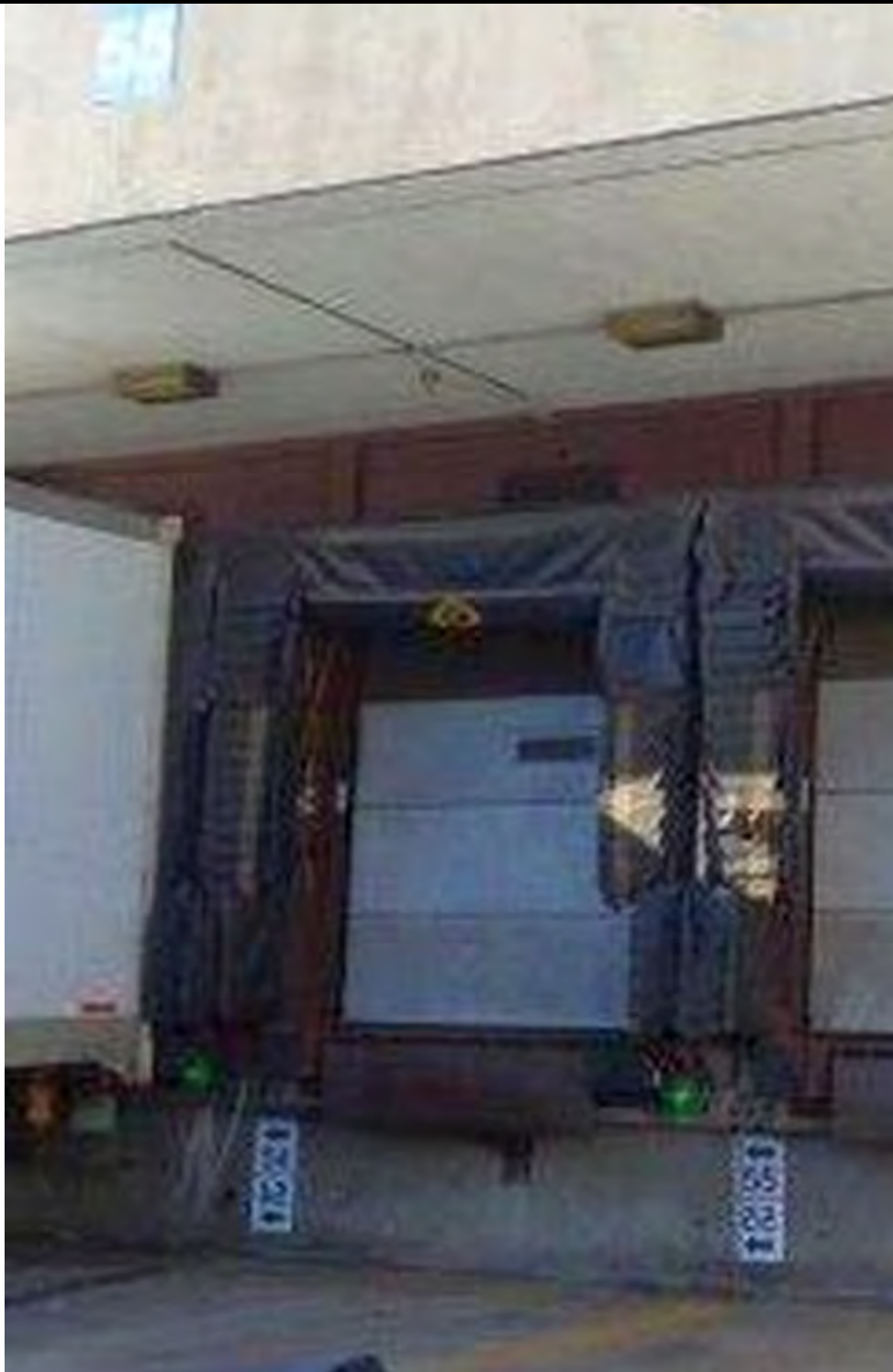
DOOR 55 Install Star 4 Truck Restraint W/ Cantilever Mounting Bracket along with Kelley Dock Control Box Mounted to Stanchion
