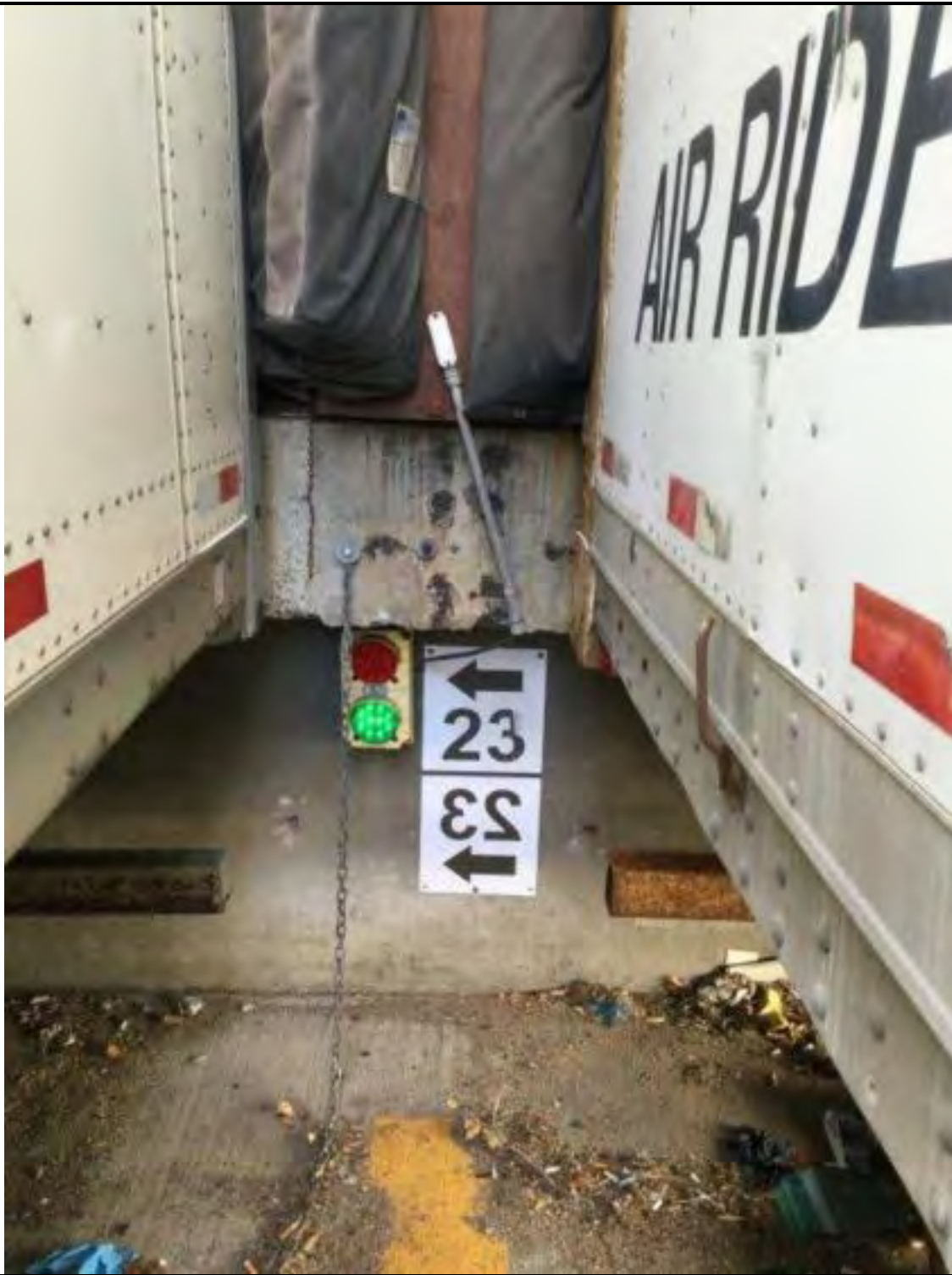
DOOR 23 Install Star 4 Truck Restraint W/ Cantilever Mounting Bracket
