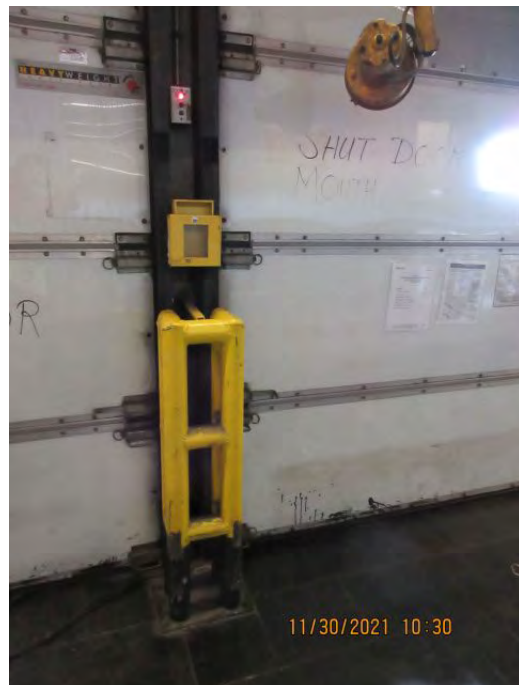
Overhead Door Control, Left side of DOOR 80
