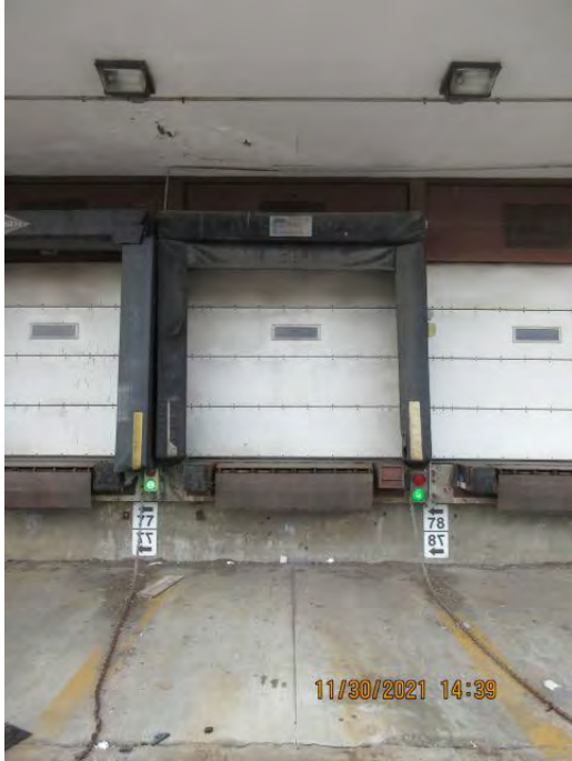
DOOR 78 Install Star 4 Truck Restraint W/ Cantilever Mounting Bracket
