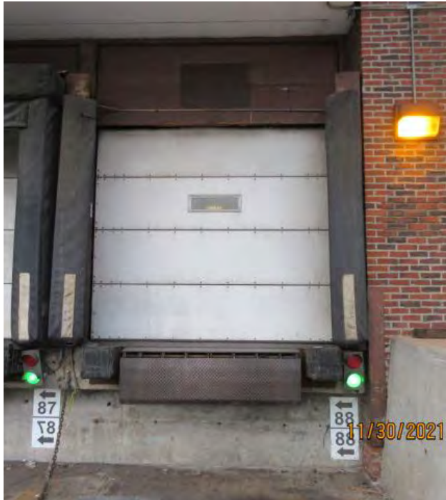
DOOR 88 Install Star 4 Truck Restraint W/ Cantilever Mounting Bracket
